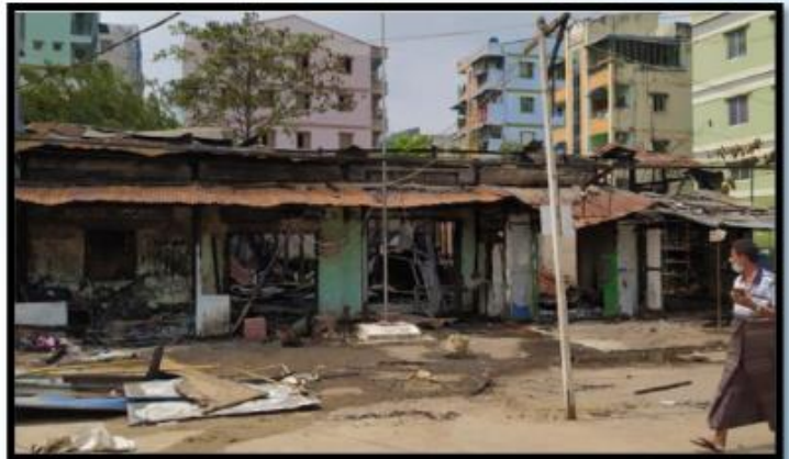
Photo 10: A ward administrative office destroyed in Yangon
